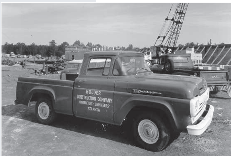
Top: "Adlers Department Store Ground Breaking." 1968. Georgia Historical Society collection of photographs. Middle and bottom: Boyle-Midway Division American Home Products Corporation construction site.
