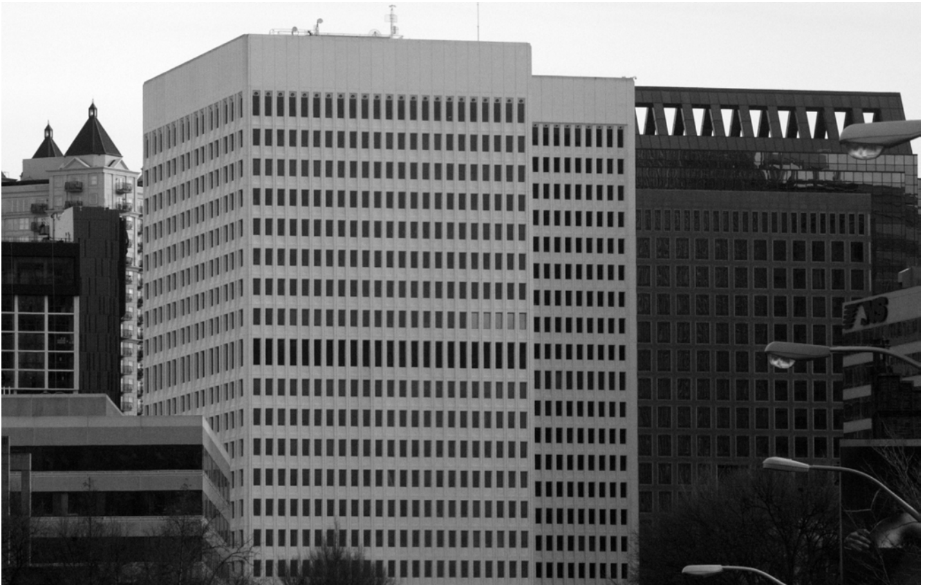
Top: Holder staff on a worksite. Bottom: Colony Square. Photo by David King.
