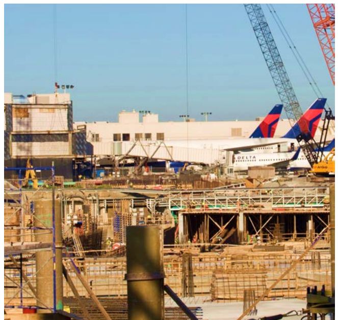
Top and right: Construction at Hartsfield-Jackson Atlanta International Airport.
