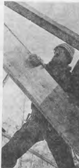
Ryan Karis supervises construction of the Visitor Center.
