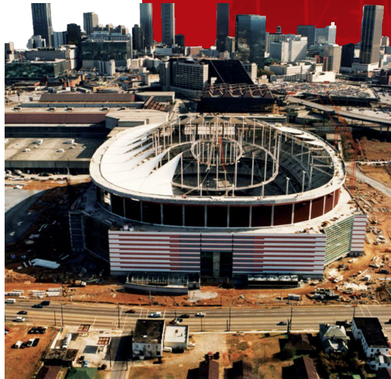
The Georgia Dome under construction in 1991.
