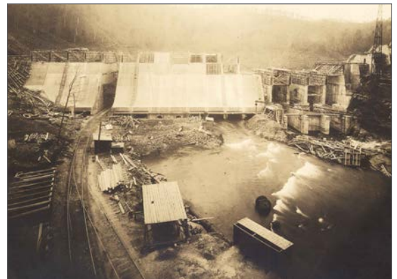
The construction of Tallulah Falls hydroelectric plant
