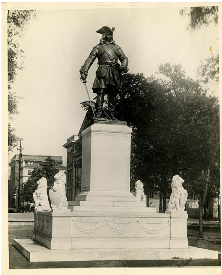
Oglethorpe Monument, Chippewa Square. From the Foltz Photography Studio Photographs. MS 1260.
